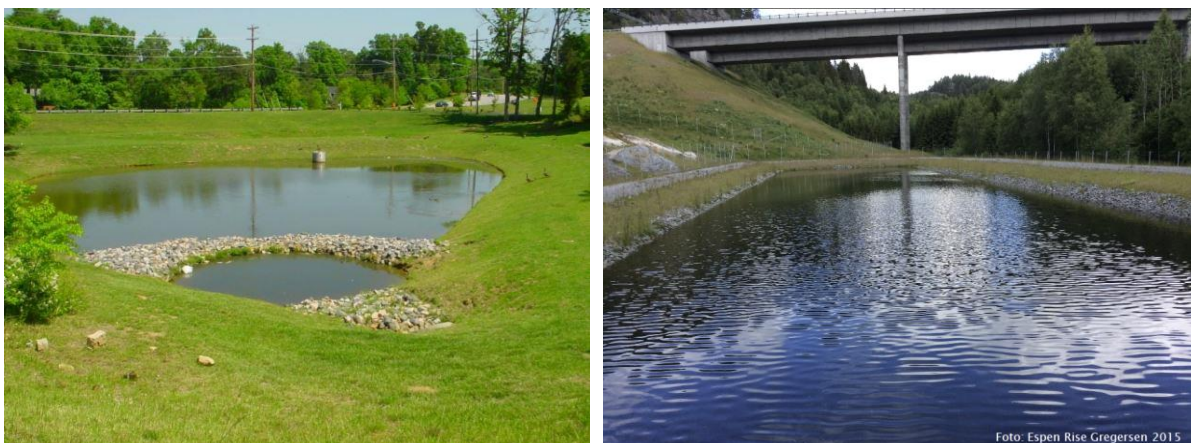
Figure 5.2 Examples of wet ponds . Left: In North Carolina (Photo: City of High Point). Right: Hobekk, E16 in Vestfold (Photo: Espen Rise Gregersen, Statens vegvesen).
