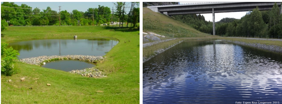
Figure 5.2 Examples of wet ponds . Left: In North Carolina (Photo: City of High Point). Right: Hobekk, E16 in Vestfold (Photo: Espen Rise Gregersen, Statens vegvesen).
