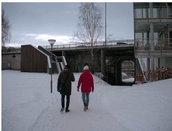
Figure 8. The elevated Klostergata is a barrier partly reduced through reopened tunnels connecting the eastern and western parts of the island of Klosterøya.
